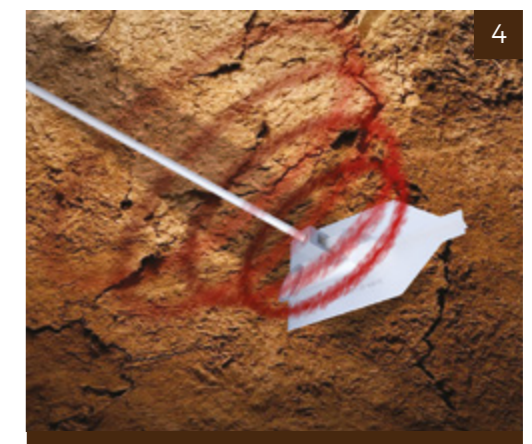
Creation of a stress zone in the shape of a truncated cone, and thereby obtaining the bearing capacity of the entire system
